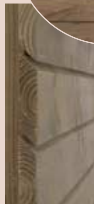
Mitered lapped planking, horizontal
