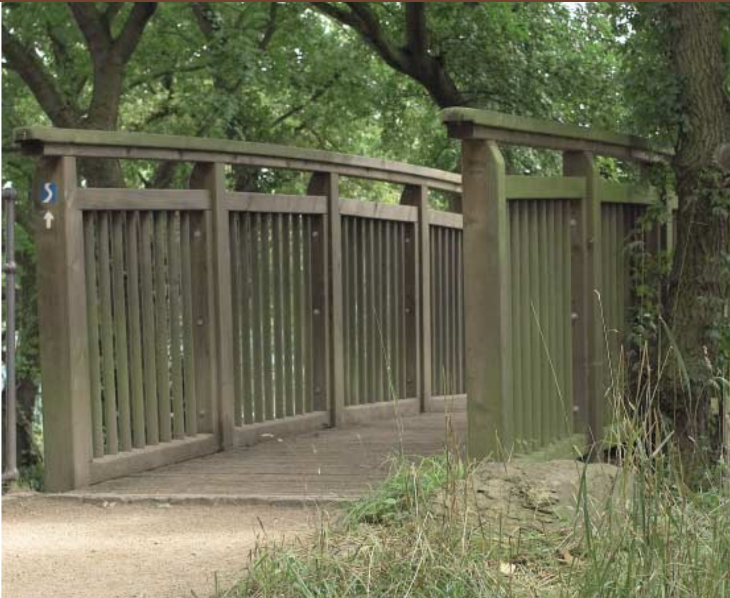
Smart construction and design suited to the landscape -- "Made by HOMBACH". Our company manufactured and built this special wooden bridge, which was installed on the plateau of the Loreley crag It bridges a ravine on the storied cliff and gives visitors a view of the breathtaking Rhein panorama.
